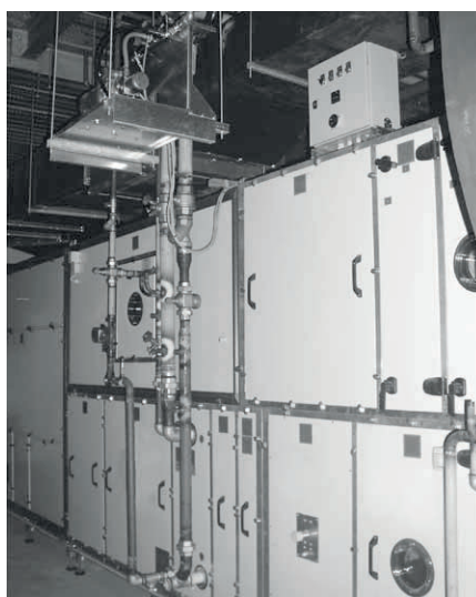
High pressure pump system
